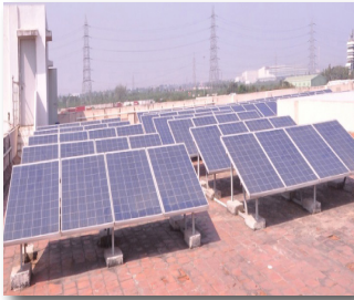
25 KW Solar Power Panel
